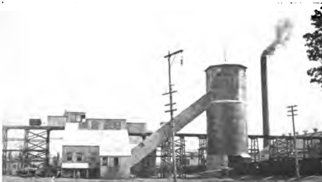
B. ROCK HOUSE AND STORAGE BIN AT AHMEEK MINE.
